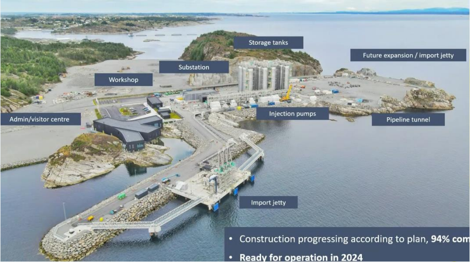
e.g. CCS Northern Lights infrastructure
