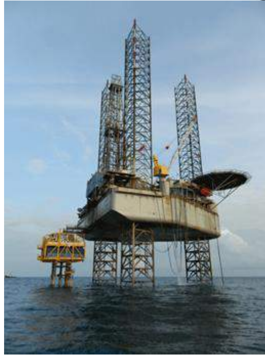
Figure 16 - Example of a Jack-up rig (Source: www.aquaterraenergy.com/the-only-way-is-jack-up-rigs-cost-effective-solutions/ ).
