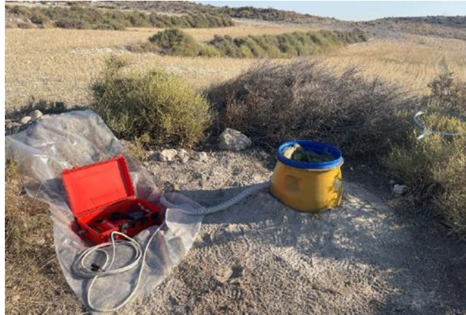
Figure 26. Datalogger installation in LOPI5. Notice the corrugated tube for the connection between sensor and datalogger.
