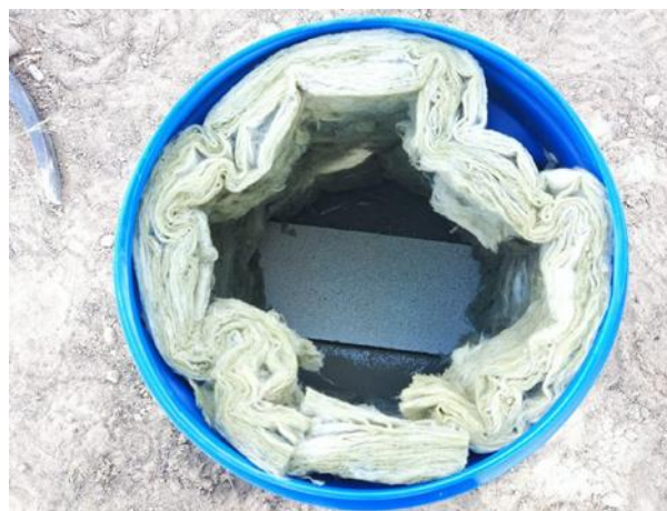
Figure 22. PVC tank, concrete slab and rock wool to thermal isolation
